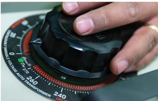
Partial Discharge Testing
